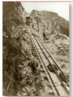
On **20 January 1890**, the first drive trial using electricity from the generator set in Maroggia was used. The experiment gave the best results and the cars covered the entire line, 1600 m, in 26 minutes.
