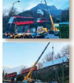
By mid-March 2024, the operation to modernise the funicular, which began in early January 2024, was completed. With an investment of over 5 million Swiss francs, the San Salvatore funicular railway has replaced not only the carriages, but also the chassis, electronics, mechanics and the haul rope.
