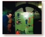
During the winter of **1982-1983** important, costly works were carried out. The company funicular staff carried out works involving consolidation along the line (sleepers and retaining walls) while the companies Kündig and Garaventa proceeded to replace the control devices and the devices for regulating the electrical drive system with a new modern electronic system. The mechanical brake control was replaced with a new hydraulic one.
