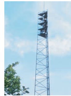
In 1950 the second 70 m lightning collector tower was erected on mount Pian San Carlo nearby.
