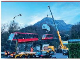
By **mid-March 2024**, the operation to modernise the funicular, which began in early January 2024, was completed. With an investment of over 5 million Swiss francs, the San Salvatore funicular railway has replaced not only the carriages, but also the chassis, electronics, mechanics and the haul rope.
