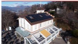
In **mid-December 2023**, the refurbishment of the Restaurant Vetta was completed. The walls were repainted, the gutters replaced, the roof renovated, and a photovoltaic system was installed on it to contribute to the restaurant's green electricity production.
