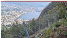
In order to protect the funicular line and the Lugano-Pazzallo district, in **November 2022**, the works to protect against the danger from falling rocks through the installation of cable-nets on the second section of the funicular have been completed with an investment of almost one million francs.
