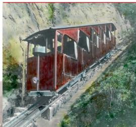
In **1938** Bell & Ci. in Kriens, Maschinenfabrik in Oerlikon and Kabelwerke in Brugg provided drive machinery ensuring greater levels of safety during operation; however this entailed changing the cable, the pinion, the drive wheels, the break pulleys and connected systems. Thanks to these modifications the driving speed increased from 1.8 m per second to 2.5 m per second, thereby reducing travel time to 14 minutes.
