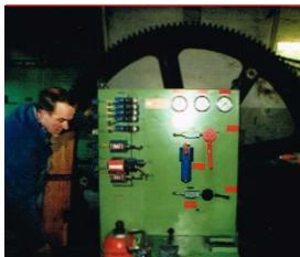
During the winter of **1982-1983** important, costly works were carried out. The company funicular staff carried out works involving consolidation along the line (sleepers and retaining walls) while the companies Kündig and Garaventa proceeded to replace the control devices and the devices for regulating the electrical drive system with a new modern electronic system. The mechanical brake control was replaced with a new hydraulic one.
